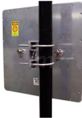
Figure 30. Installing Flat Panel Antenna to the Pole
