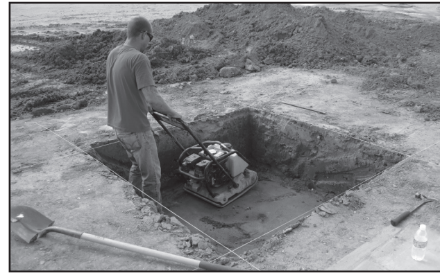
Soil Density compacted to 95% per ASTM-698
