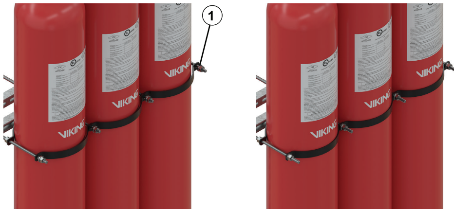
Figure 6.7: Tighten brackets
