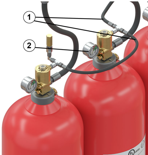
Figure 12.3: Removing the pneumatic pilot lines
