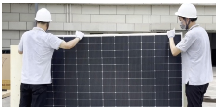
5.1.3.13 After removing the module, slowly turn it to horizontal position and placed it on transport racks. When stacking, ensure junction boxes and connectors are staggered and never stack more than four modules.
